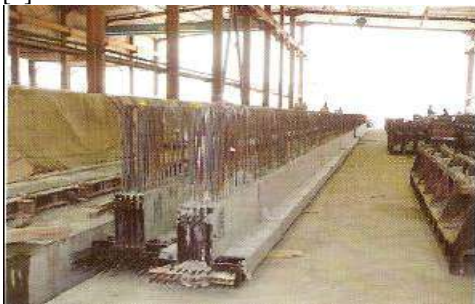
Figure 1 Manufacturing of Precast members in controlled environment i.e. in factory [14]
