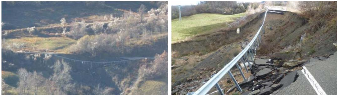
Figure 3: Details of the street interruption in sector G3 (November 2010).
