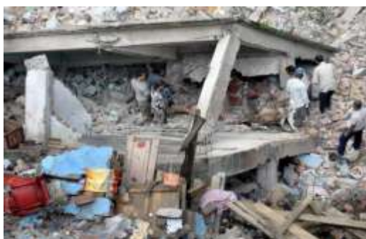
Fig. 11 Column failure during Nepal Earthquake [11]
