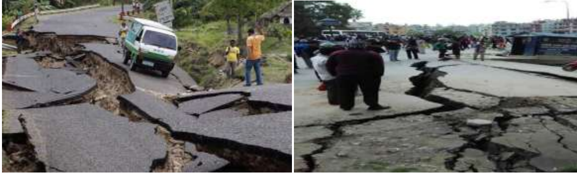
Fig. 7 A huge cracks have opened up in this road after the Nepalese capital was rocked by a 7.8-magnitude tremor [11]
