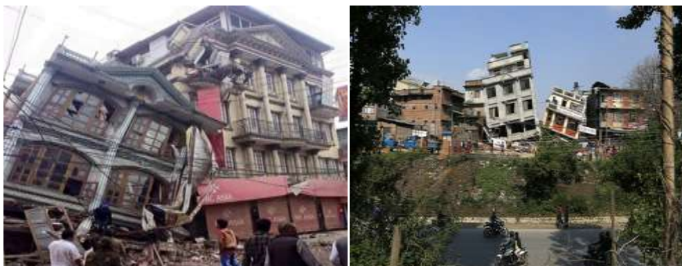
Fig. 9 Building deflects due to pounding effect during earthquake vibrations [11]
