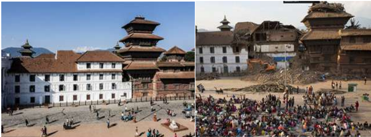
Fig. 3 People gather in Durbar Square for security reasons. Complete masonry failure [1]
