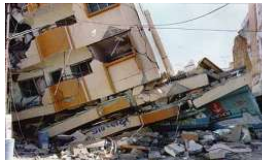
Fig. 8 Collapse of soft storey [11]
