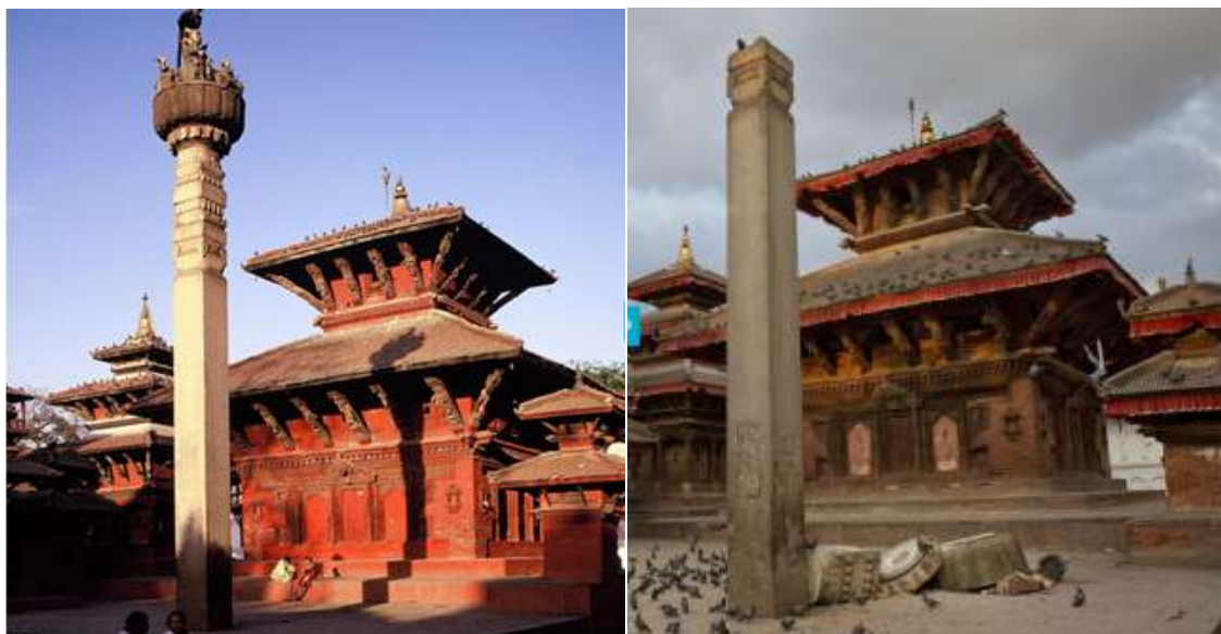
Fig. 6 Failure of minaret due to poor construction [11]
