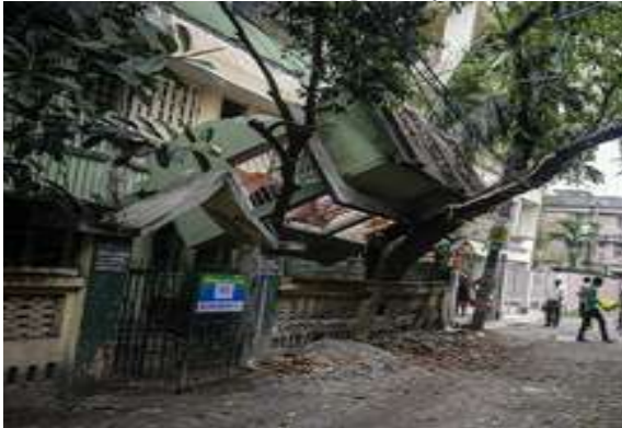
Fig. 10 Balcony of the building toppled [11]
