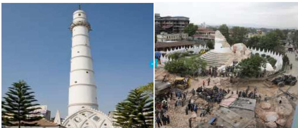
Fig. 4 The Iconic Bhimsen Tower before and after the earthquake [1]
