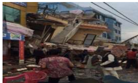
Fig. 13 Twisting of building during Nepal Earthquake [11]
