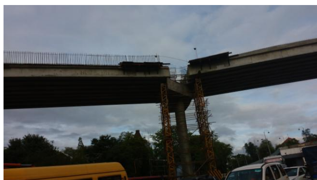
Image 2.Flyover Construction at site
