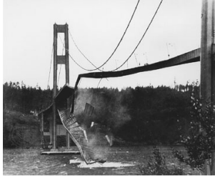
Figure 1: Collapse of the Tacoma Bridge [4].
