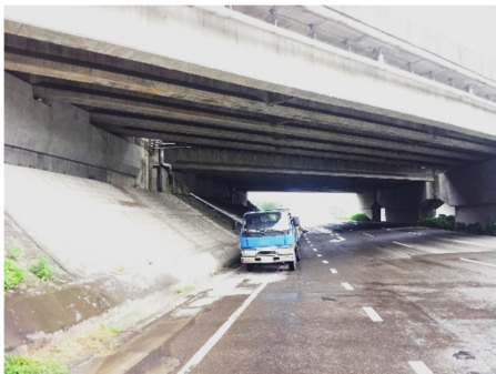
Fig. 5. Freeway overpass with significant levels of ground noise
