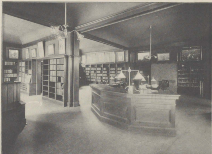
INTERIOR OF DARLINGTON LIBRARY
