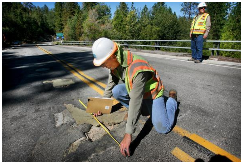
Figure 1. Human conducted visual inspection with simple equipment [6].
