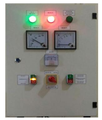
Figure 2. Automatic transfer switch operation on PLN electricity and power inverters
