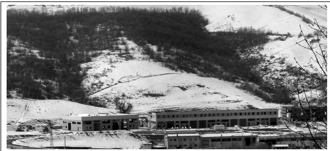
Fig. 4 – Industrial buildings recently constructed at the foot of the Ca' Bonettini landslide (March 2004)
