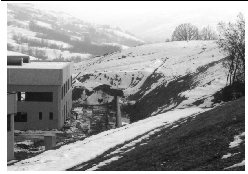
Fig. 5 – Slope cut at the foot of the Ca' Bonettini landslide and containment wall (March 2004)
