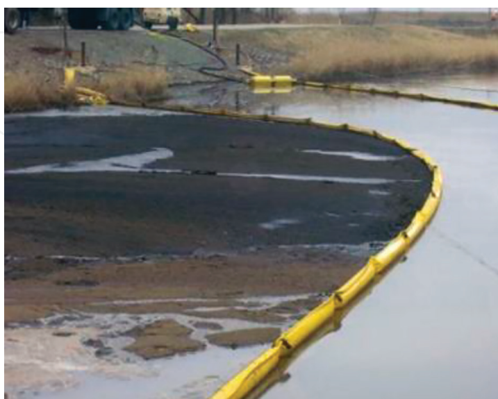
Figure 3. Use of the oil containment boom [28].
