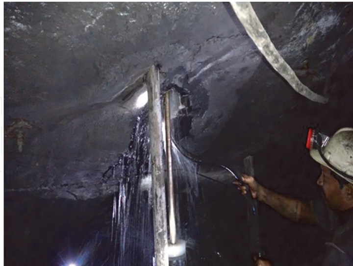
Figure 24. Drilling of EX size borehole (Pilot hole).
