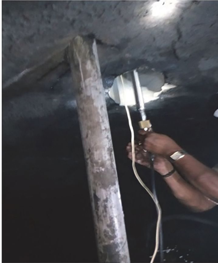
Figure 28. Installation of CISRO HI cell.
