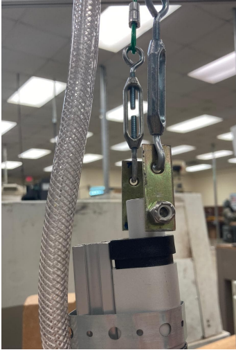
Figure 9. Mechanical Cables with Actuator
