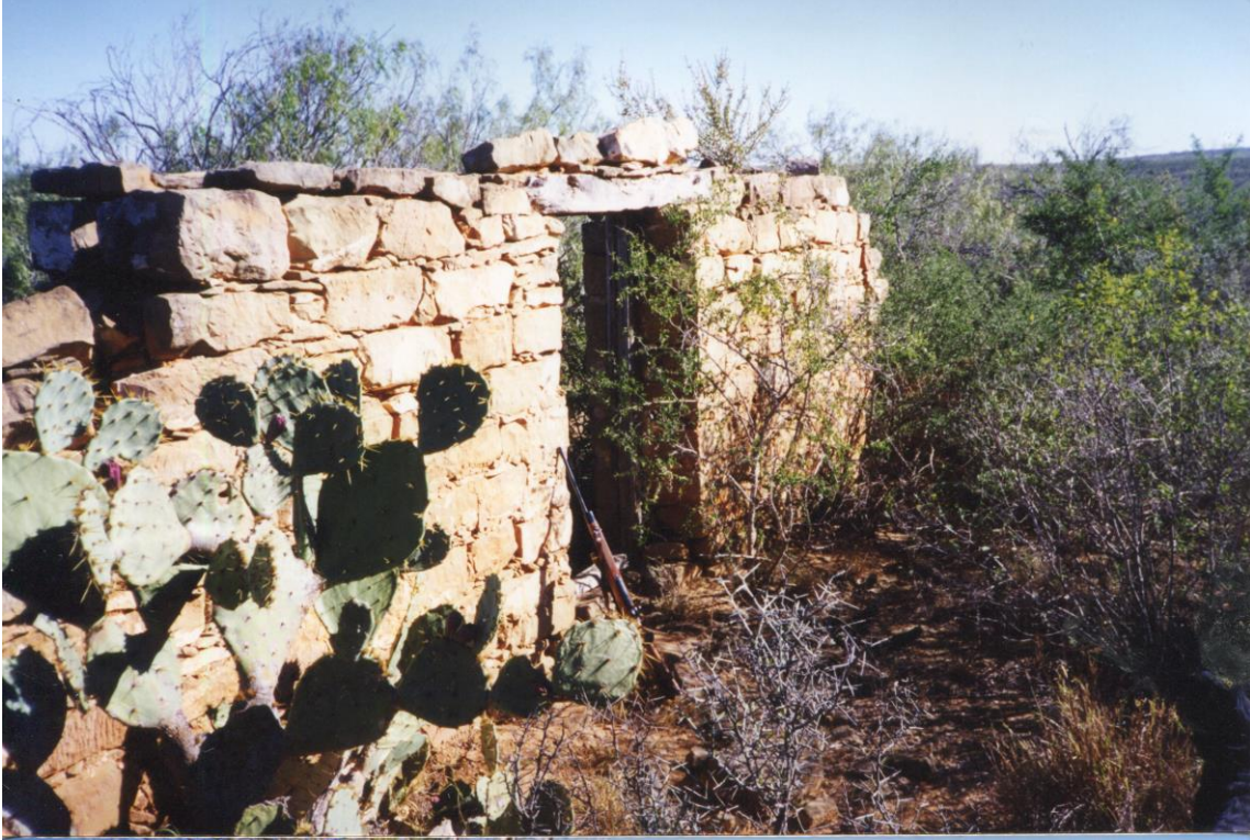
Sandstone structure in ruins.
