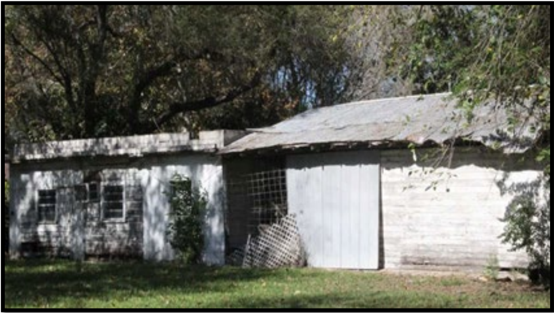
Figure 5.1 Bracero Quarters on the Luna Farm property
