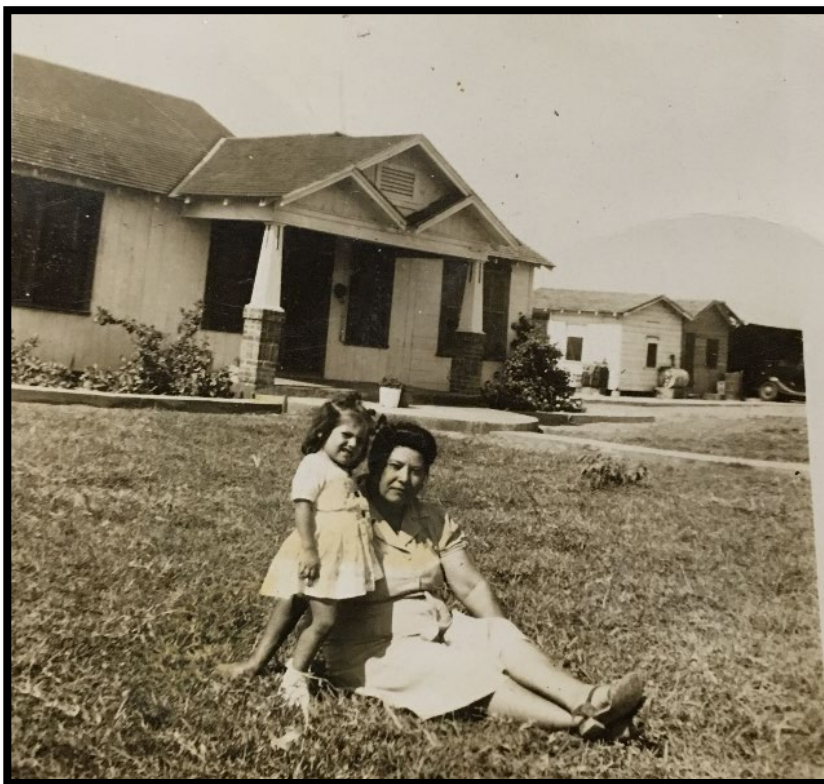
Fig 4.2 Maria G. Luna and Teresa: Second home moved closer to infrastructure.
