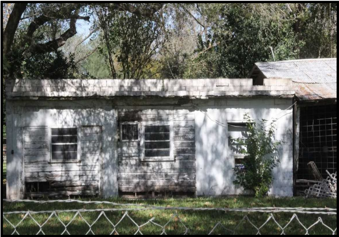
Figure 5.1 & 5.2 The Bracero's former quarters on the Luna family farm
