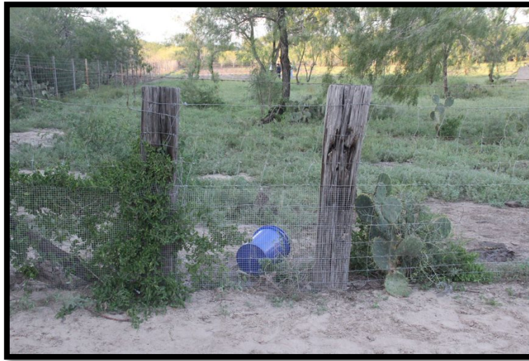
Figure 3.27 Original mesquite end-posts on Janie's property near the rear.
