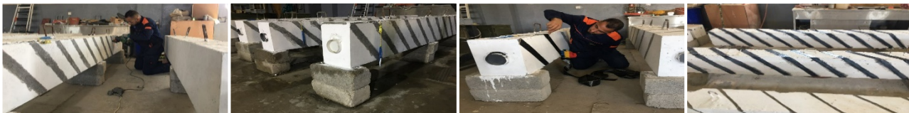
Fig. 4. Applying the CFRP system to the concrete beams.
