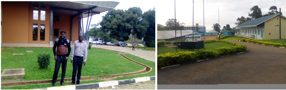
Picture 1.7. Technical and vocational teacher education block, Kyambogo University. Fisheries Training Institute (FTI) Classroom blocks.
