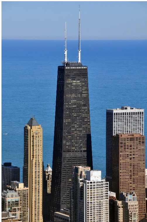
Figure 3 875 North Michigan Avenue (Wikipedia)
