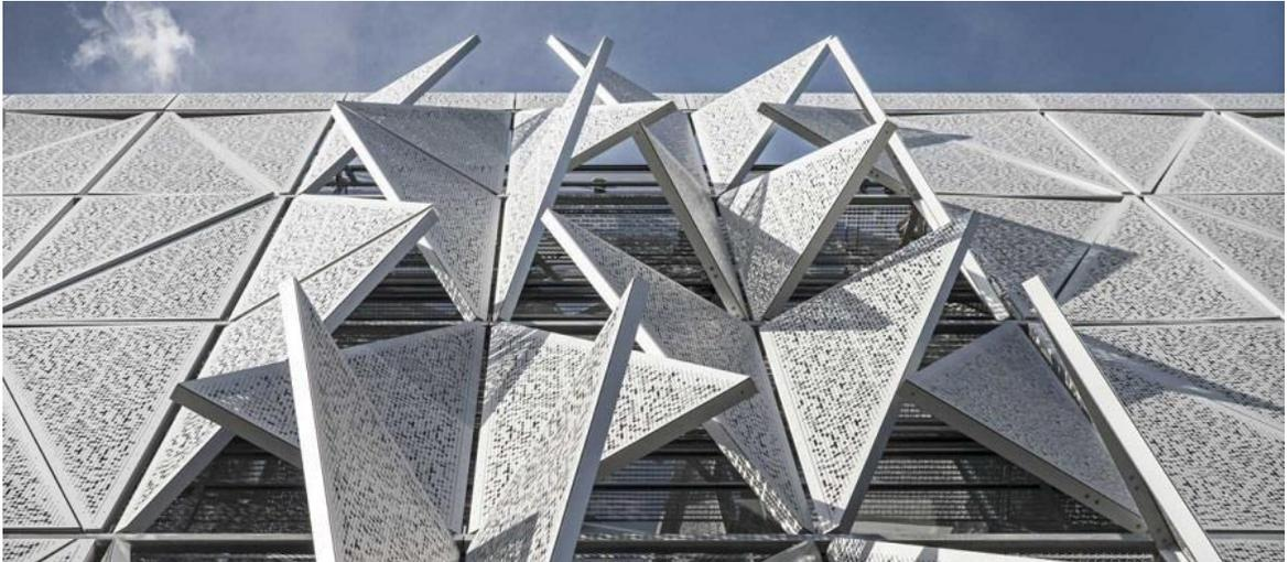
(Figura 9.15.) Sistema cinético de la fachada del Kolding campus. Recuperado de: <https://www.e-architect.co.uk/denmark/kolding-campus-university-southern-denmark> el 17/11/20
