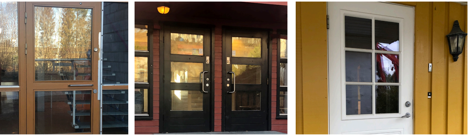
Examples of exterior doors. Photo: SINTEF Community
