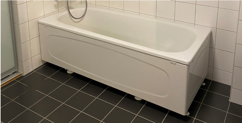
Examples of bathtubs in enameled steel with removable skirt. Photo: SINTEF Community
