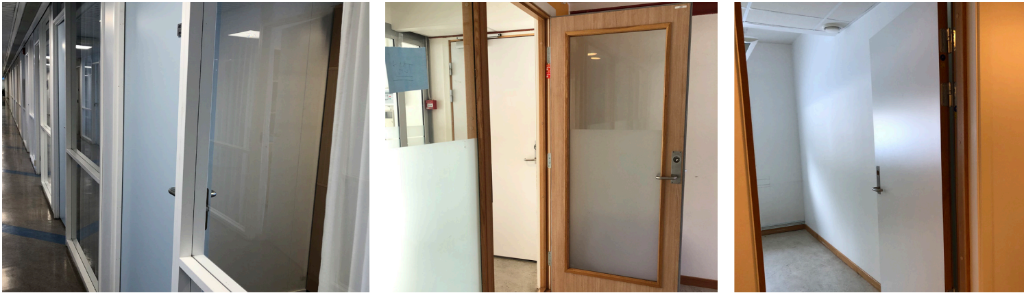
Examples of interior doors. Photo: SINTEF Community
