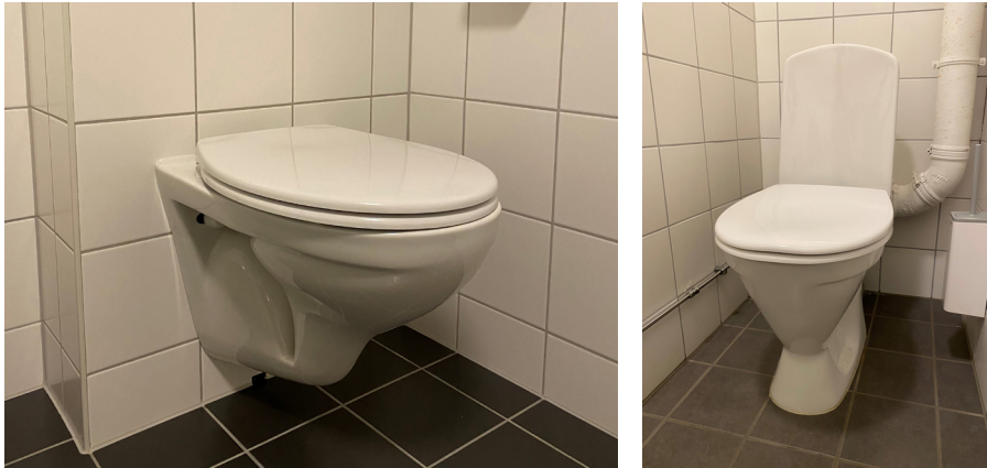
Example of a wall-mounted WC suit (P-trap) and a floor-mounted WC suit (S-trap) with cistern. Photo: SINTEF Community
