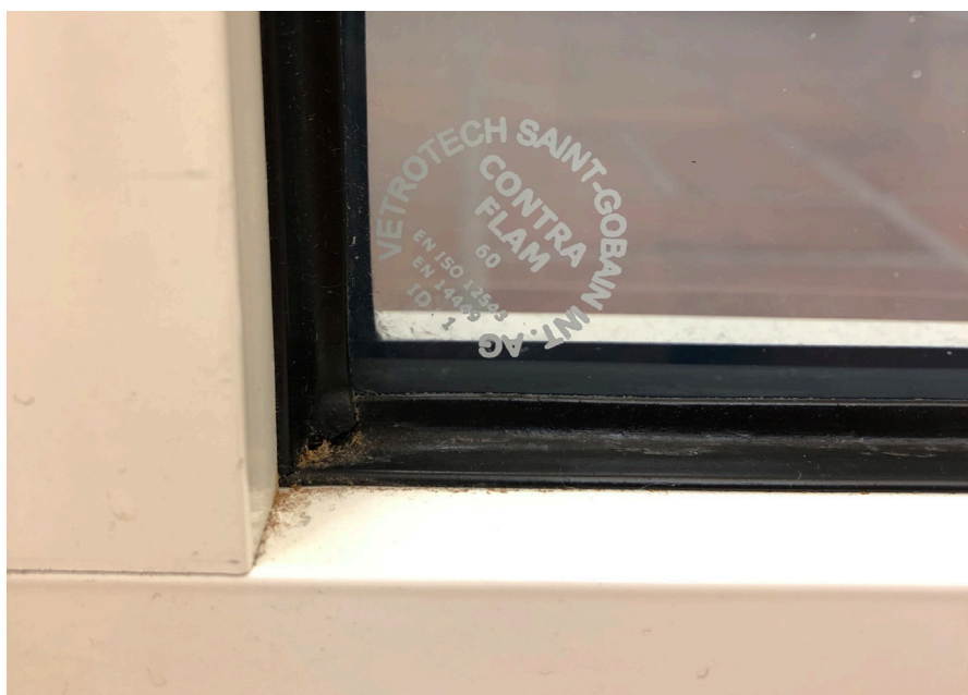
Example of labelling on interior glass walls. Photo: SINTEF Community
