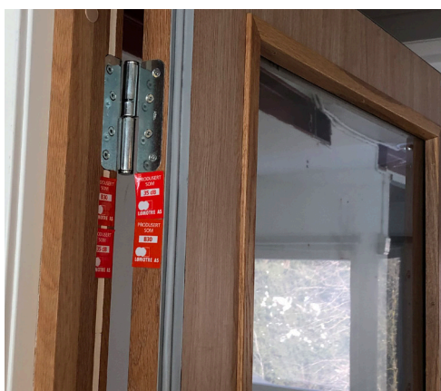
Sound insulating or fire resistant properties are often indicated by labelling on the frame or outer edge of the door. Photo: SINTEF Community
