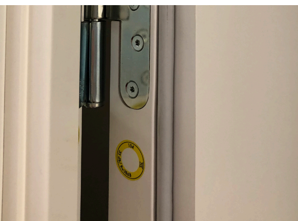
Sound insulating or fire resistant properties are often indicated by labelling on the frame or outer edge of the door. Photo: SINTEF Community
