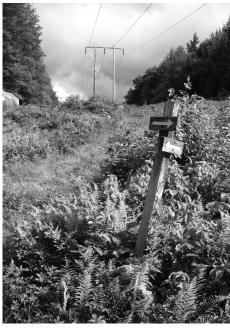
Wooden towers about 50 feet tall historically have carried power through the White Mountain National Forest. Hydro-Quebec's proposed Northern Pass towers would replace these towers with a parallel set of 85-foot-high steel monopole and lattice towers that would exceed tree height across 10 miles of the WMNF. APPALACHIAN MOUNTAIN CLUB
