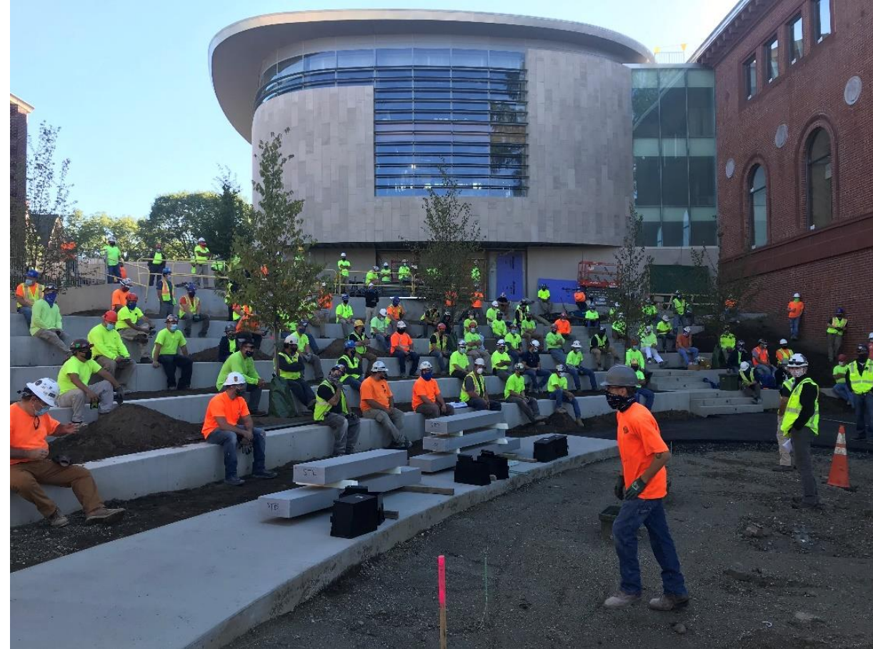
Safety Meeting, Photo credit: Shawmut Design and Construction
