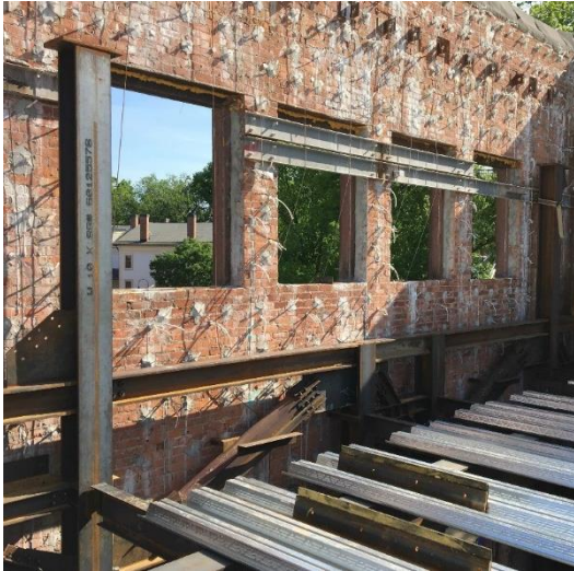
Thermal break between old and new
