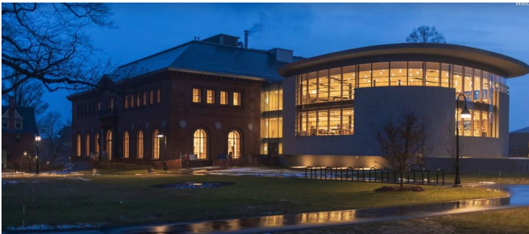
30% window-to-wall ratio supports energy goals
