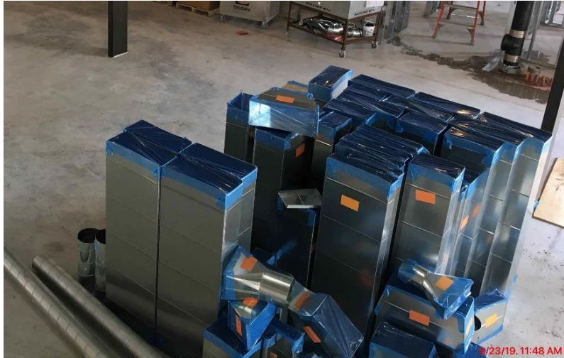
Covered ductwork during construction, Shawmut
