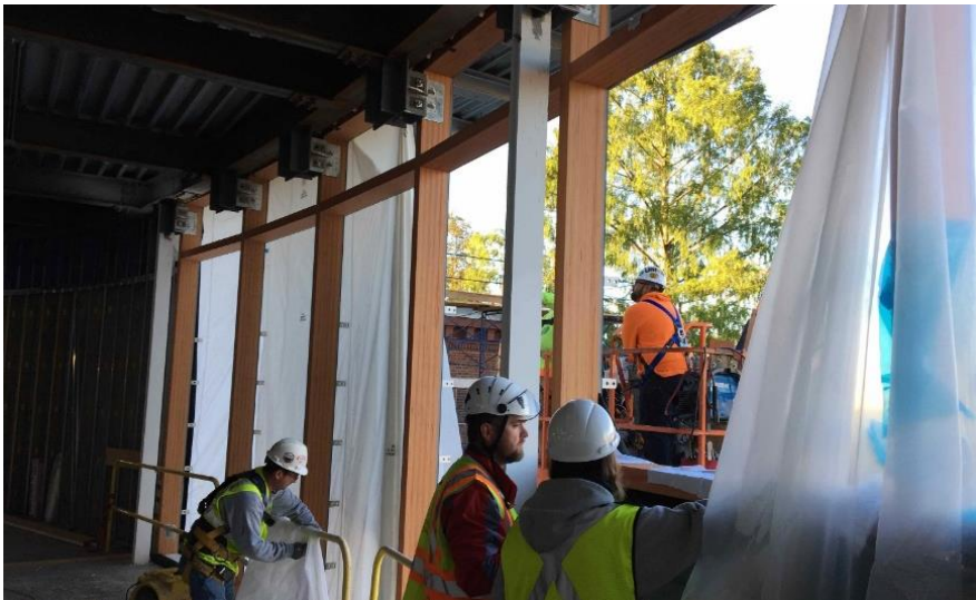
Images highlighting the timber-framed curtain wall.
