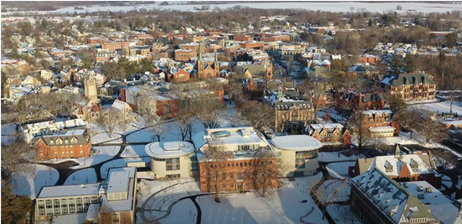
Image capture: Smith College, The New Neilson Video Tour March 2021
