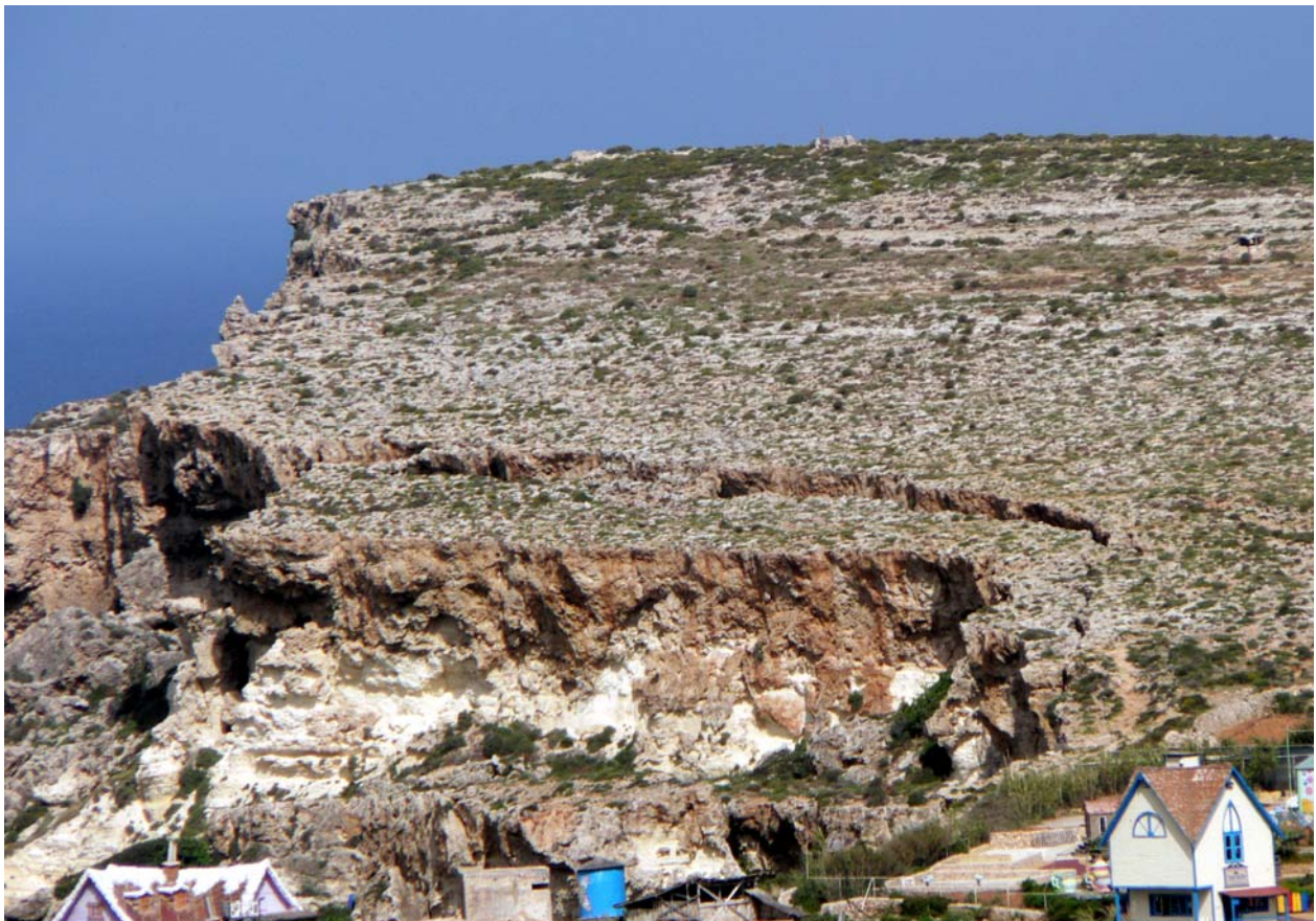
Fig.18: Lateral spreading at Anchor Bay.
