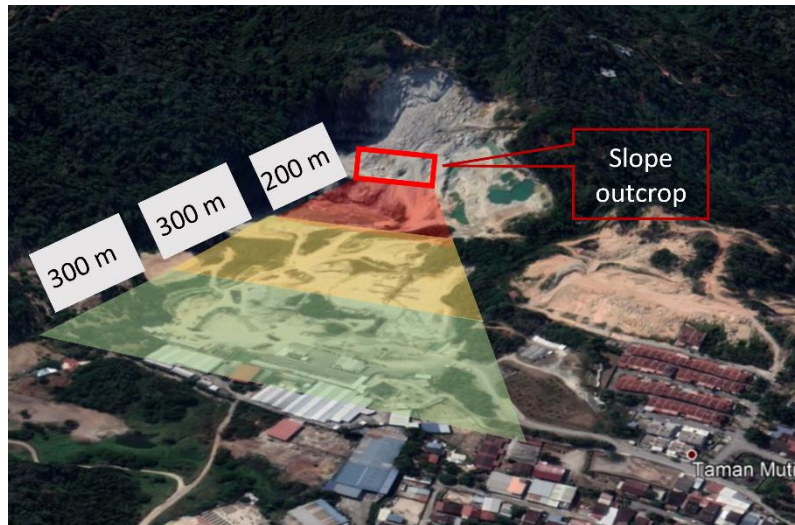
Fig. 5 - Proposed georisk zoning for rock slope failure hazard
