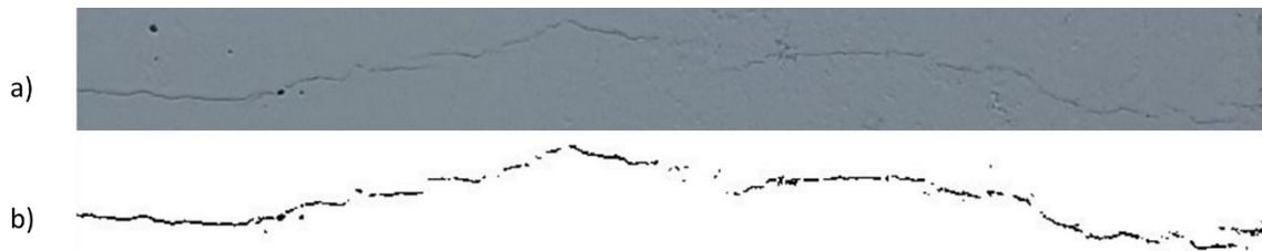
Figure 39. Crack segment analysis: a) duplicate of crack segment selection, and b) isolated crack after 8-bit conversion and threshold adjustment of a crack segment
