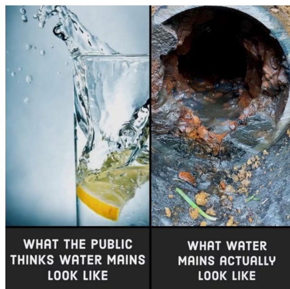
Figure 1-1. A Typical Deteriorated Water Main under Service (Source: Murphy Pipeline Contractors, https://www.murphypipelines.com/ )
