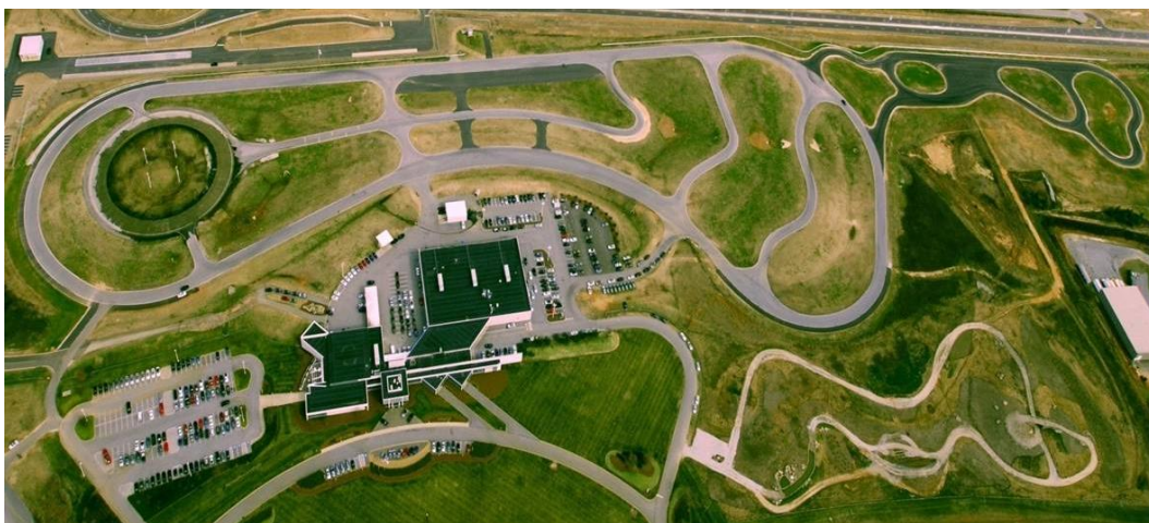
Figure 24. Aerial view of the closed-road course.
