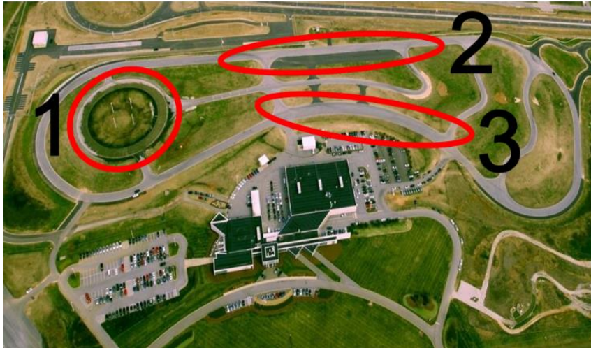
Figure 10. Aerial view of the track with the locations of the 1 ABS braking, 2 skid recovery, and 3 distraction exercises indicated.
