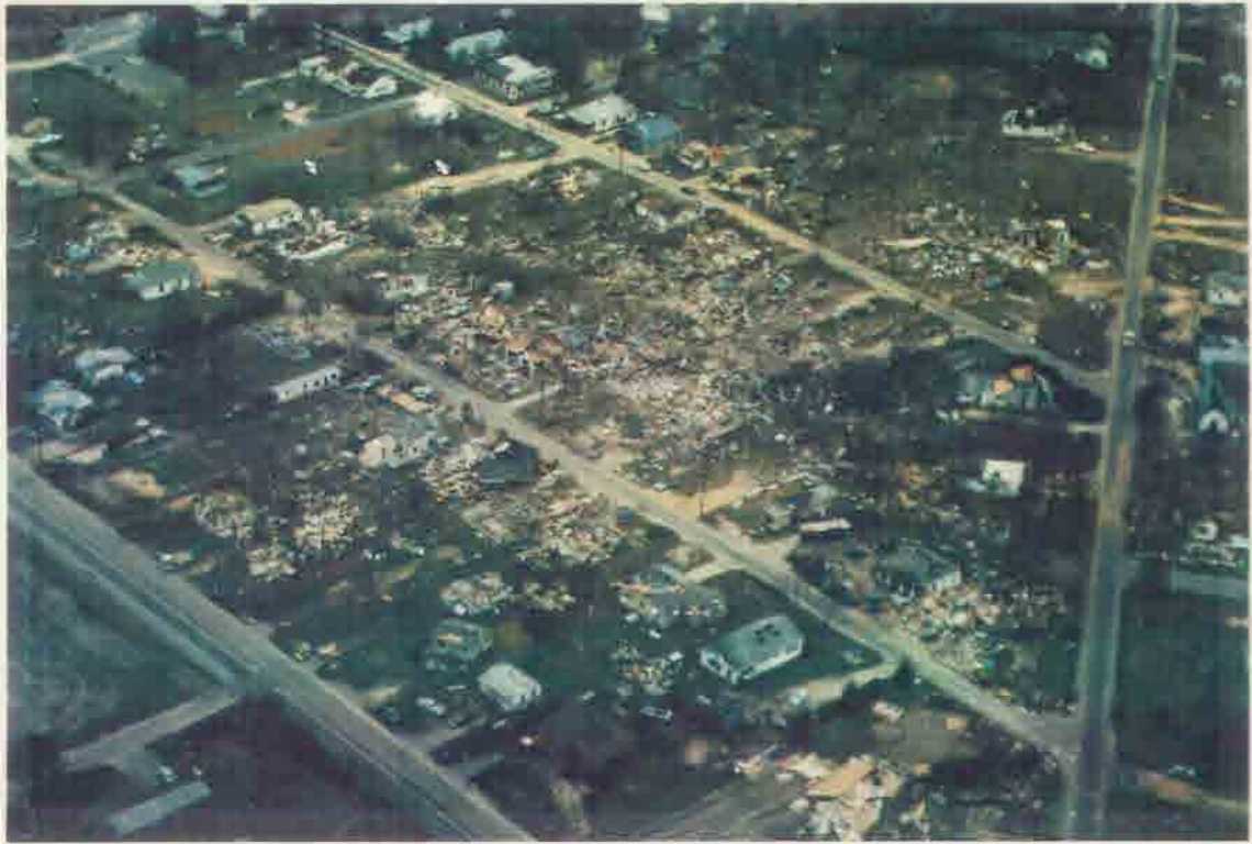
Fig. 1 Photograph from aircraft of damage done by a tornado in North Carolina during the 28 March 1984 outbreak.
