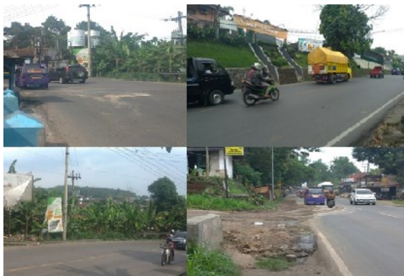
Figure 10. Existing Condition of STA 1
