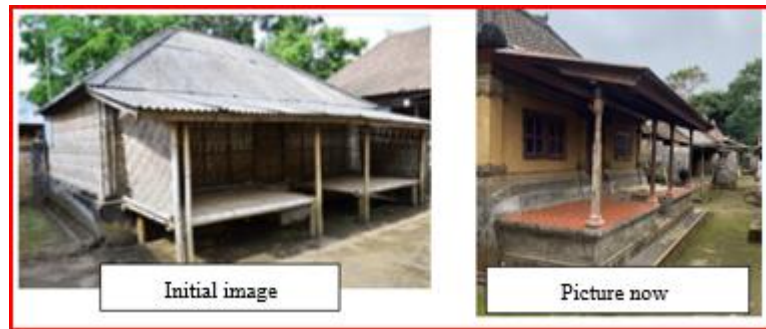
Figure 23. Modernization of Bale Meten (Results of analysis, 2022)
