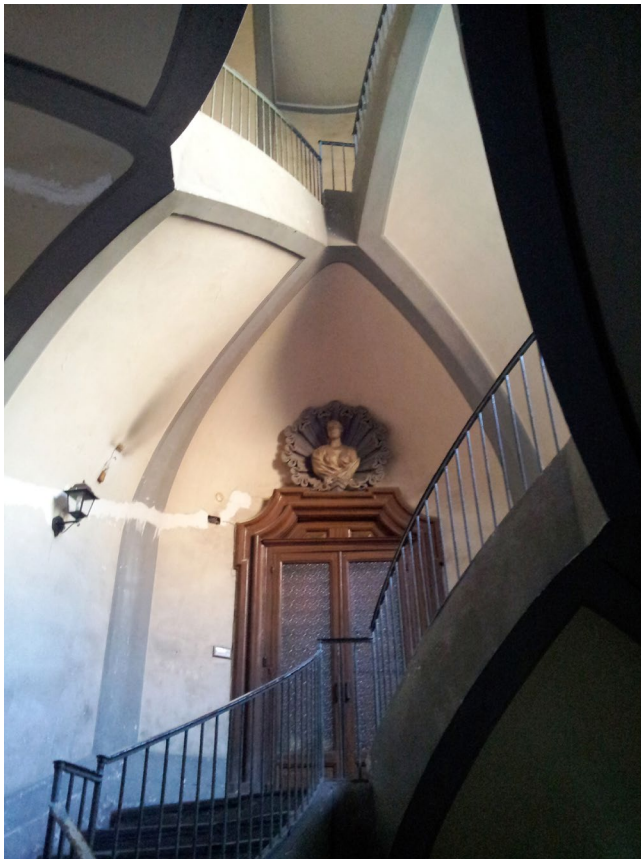
Figure 9. Palazzo Di Majo's staircase: development of the staircase from one of the balconies, with a view from below of the vaults forming the ramps and landings. Picture by the authors.
