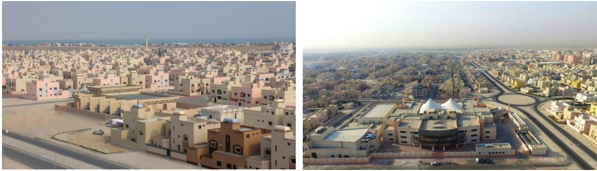
Figure 1 Jaber Al Ahmad City Housing Project (cgtm.com. 2019)
