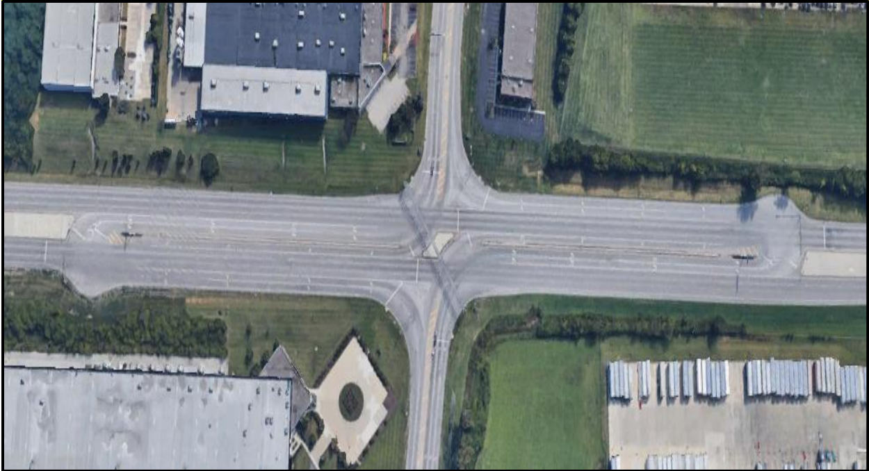
Figure 3.3: RCUT intersection at OH-4 Bypass and Symmes Rd, Hamilton, OH ( Google Earth )
