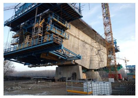
FIGURE 12. Balanced cantilever under construction at pier D2.
