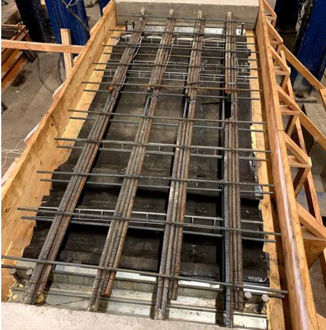
Figure 10.17: Completed Link Slab Reinforcement
