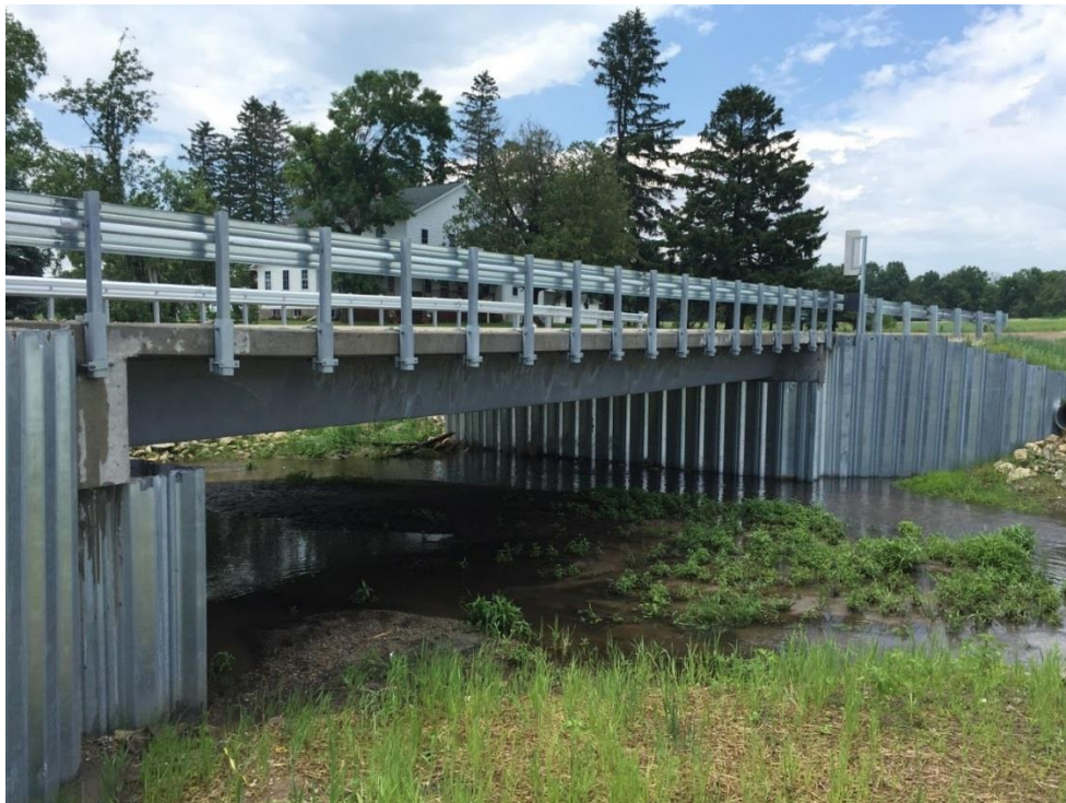
Figure 2.20: New Amish Sawmill Bridge (Gibbs, 2017)
