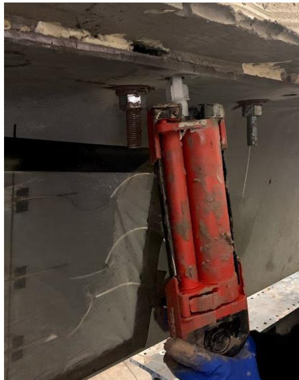
Figure 10.25: Hilti HIT-HY 200-R Adhesive Injection
