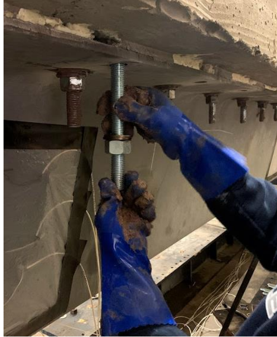
Figure 10.26: Insertion of Threaded Rods with a Twisting Motion
