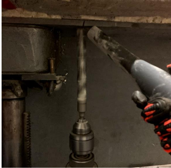
Figure 10.24: Concrete Drilling with Wet and Dry Shop Vacuum to Control Dust
