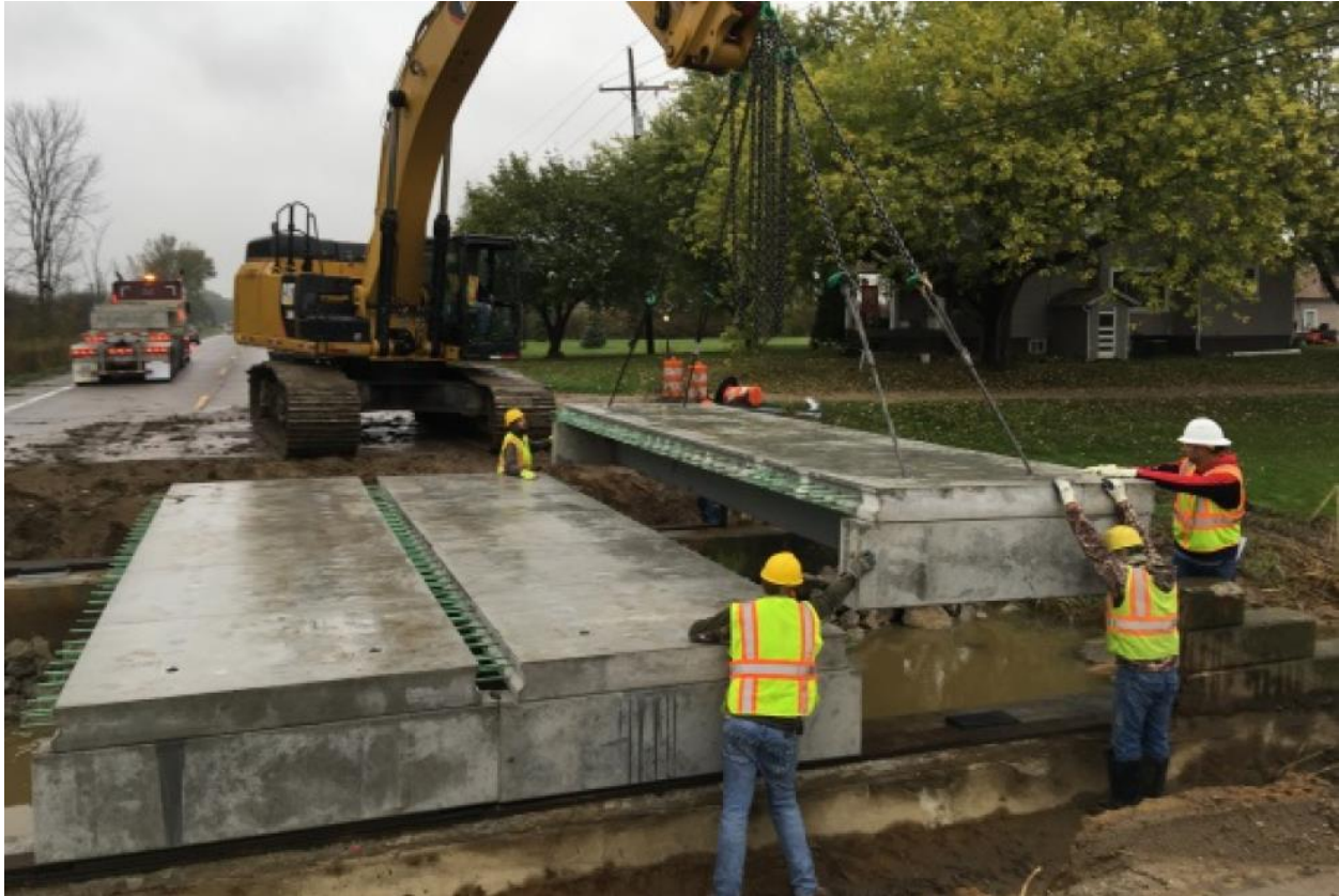
Figure 2.8: Superstructure Placement of Composite Modules (SSSBA, 2021)
