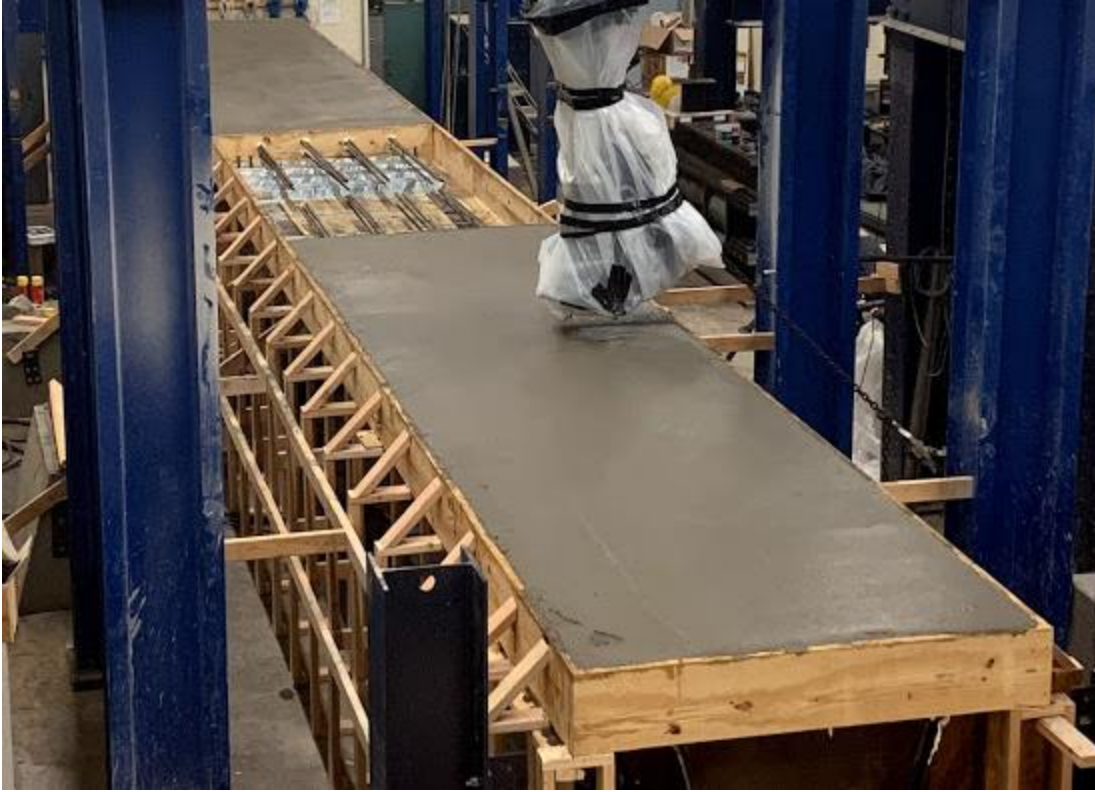
Figure 10.15: Finished Main Span Concrete Decks
