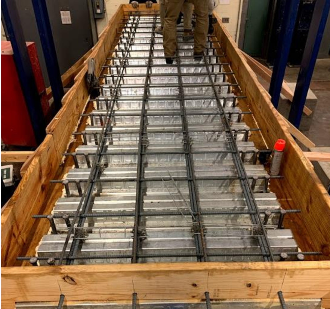
Figure 10.13: Placement of Concrete Deck Reinforcement
