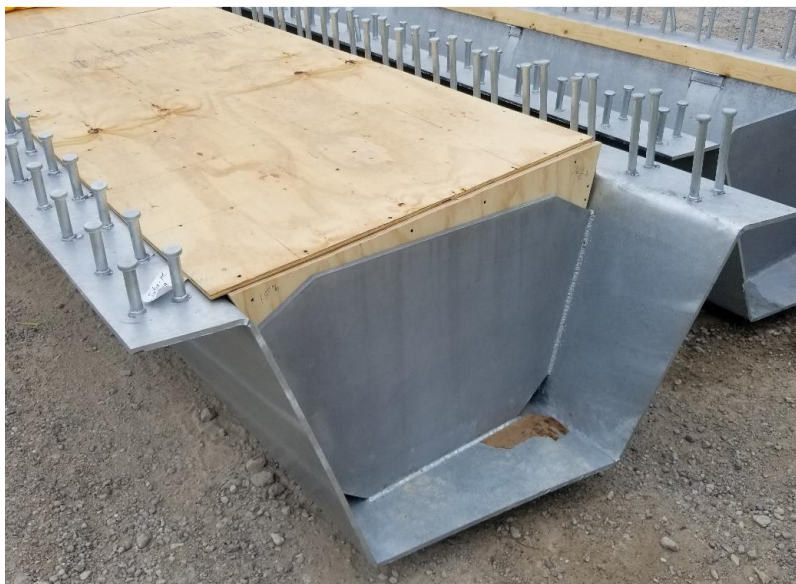
Figure 2.23: PBFTG with Completed Internal Formwork (Roh, 2020)
