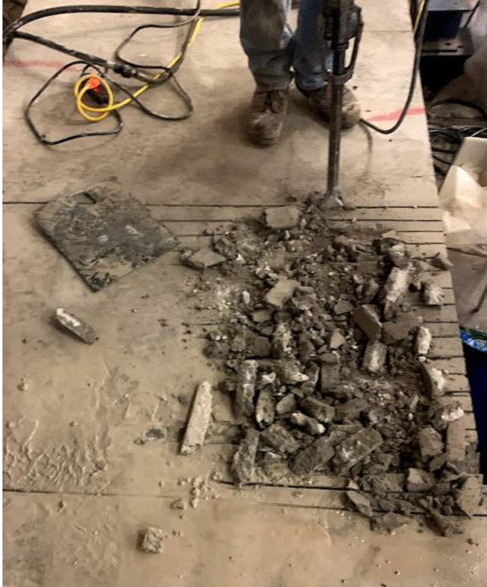
Figure 10.29: Concrete Deck Removal
