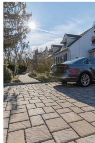
CO 2 -cured Solidia Concrete™ from EP Henry Newark, DE
