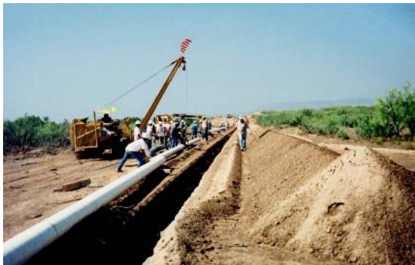
Figure 5-10: The 10-inch Diameter Val Verde Pipeline Transports CO 2 from Four Gas Treating Plants to the Canyon Reef Carriers Pipeline, Used for EOR Operations 56
