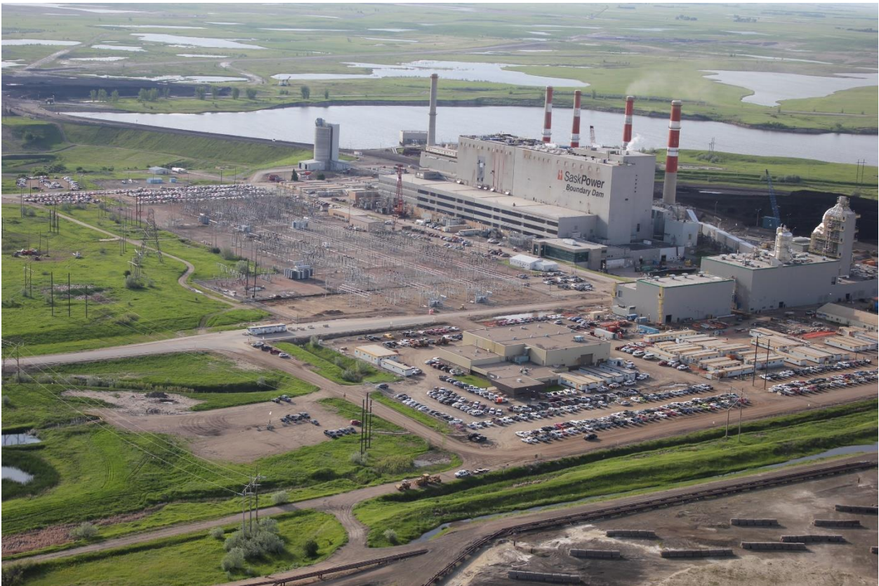
A World's First: Boundary Dam CCS Project (Image credit: SaskPower)
