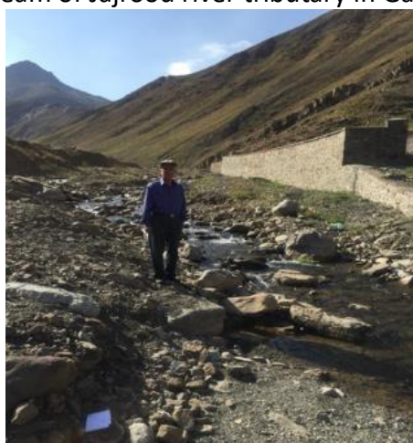
Figure 3 - Upstream of Jajrood river tributary in Garmābdar region.
