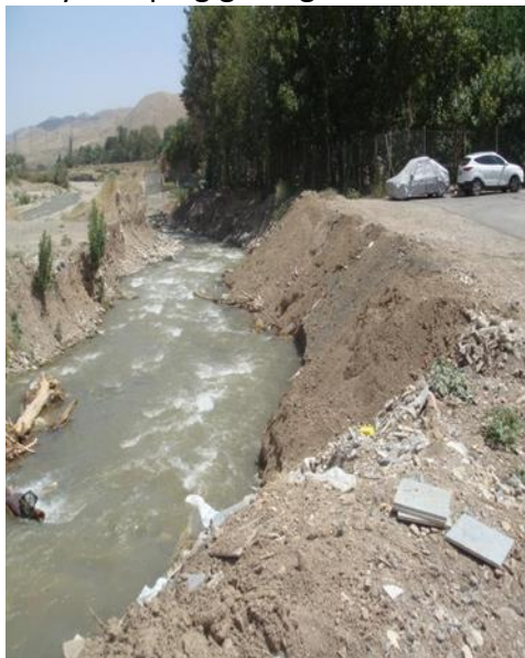
Figure 12 - Effects of tree trunks and destruction of river banks due to floods in 2018 and unfortunately dumping garbage into the river channel.
