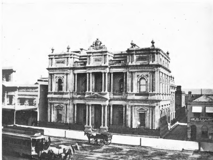
South Australian State Archives, Adelaide The land for this building on the west side of King William Street was bought by the Bank of South Australia in 1866, the contract was let in 1875, and in June 1878 the Bank moved there from North Terrace.
