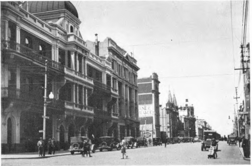
Government Printing Office, Perth 84 St. George's Terrace, 1922. The offices of the Union Bank of Australia are the four-storey building this side of the vacant land.
