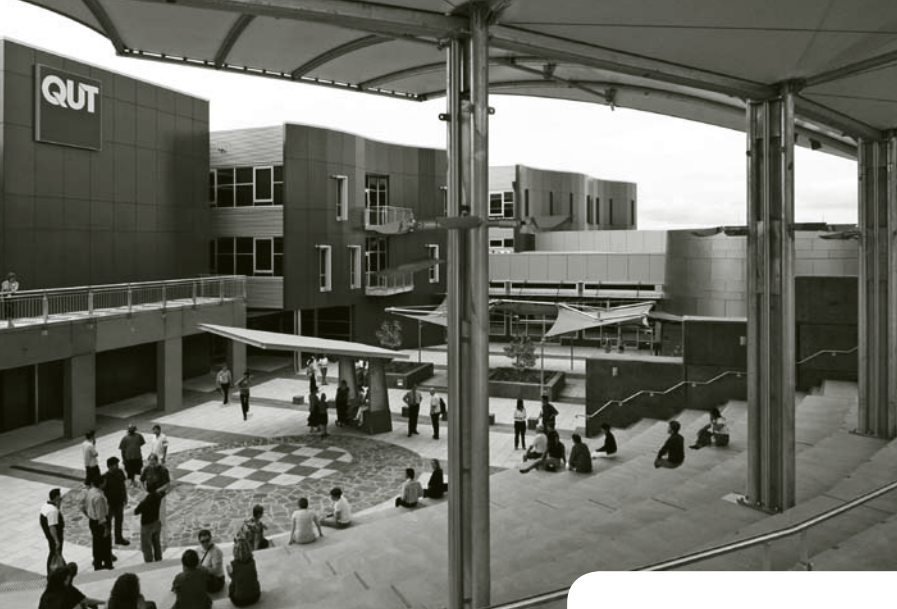
The new Student Learning and Support Centre at Kelvin Grove brings together learning facilities for students and accommodation for student support staff.
