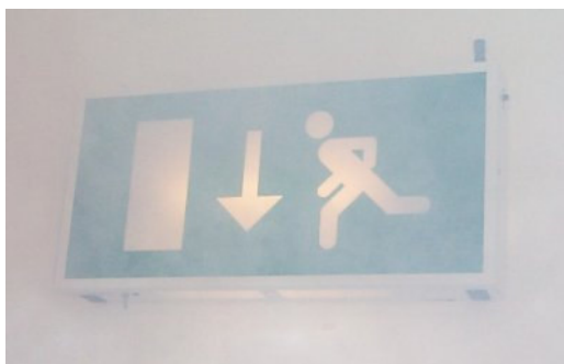
Figure 6.2 Smoke obscured exit system
