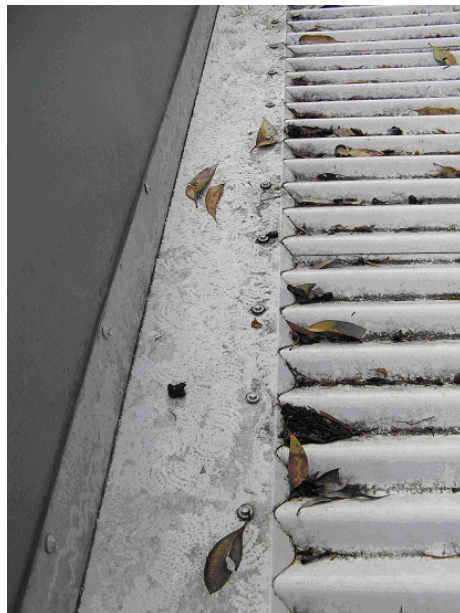
Figure 3.16. Flashing between wall and roof.
