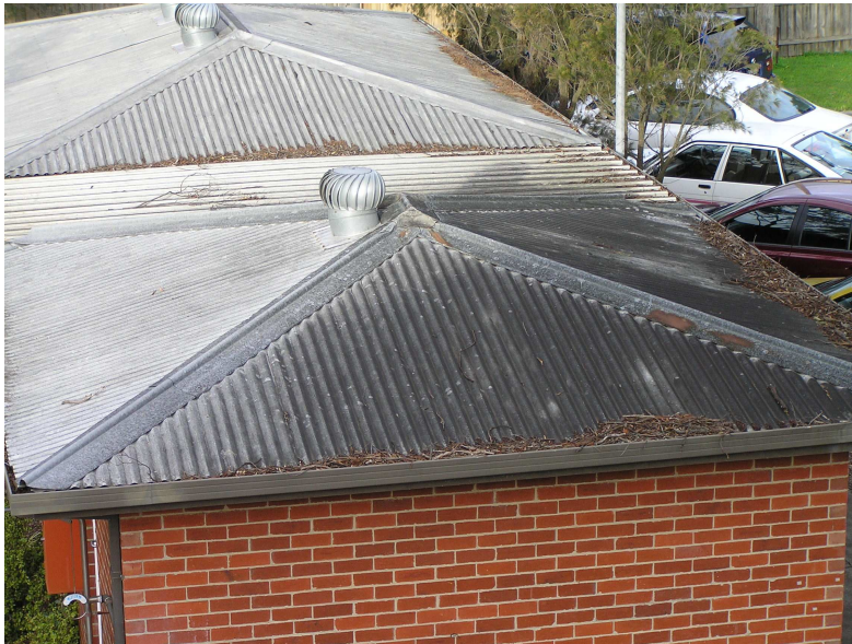
Figure 3.15. Illustration of metal ridge capping.
