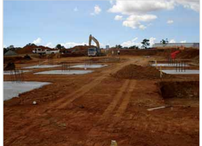
JCC site at start of construction
