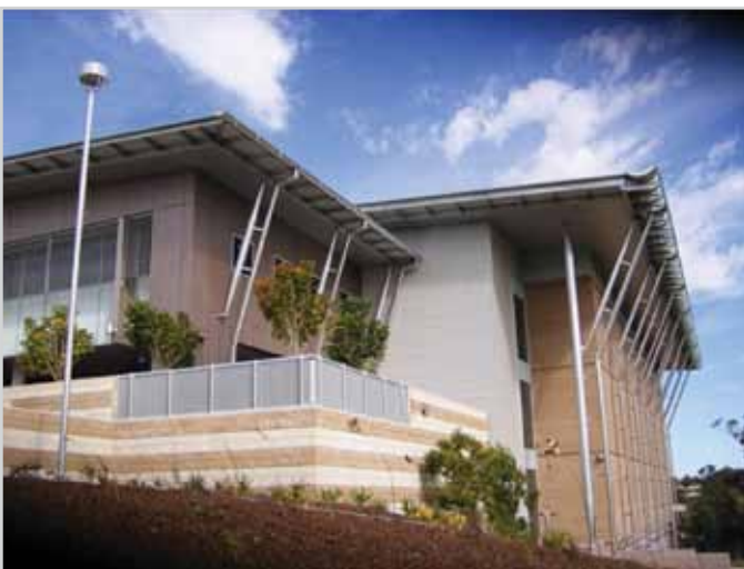
State Archives Extension Project after practical completion, September 2008
