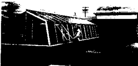
Figure 1.—Compartmented greenhouse used for production of sugar-beet seed at Salinas, California. Filtered air from fan house (top, right) is supplied to each chamber through underground ducts.
