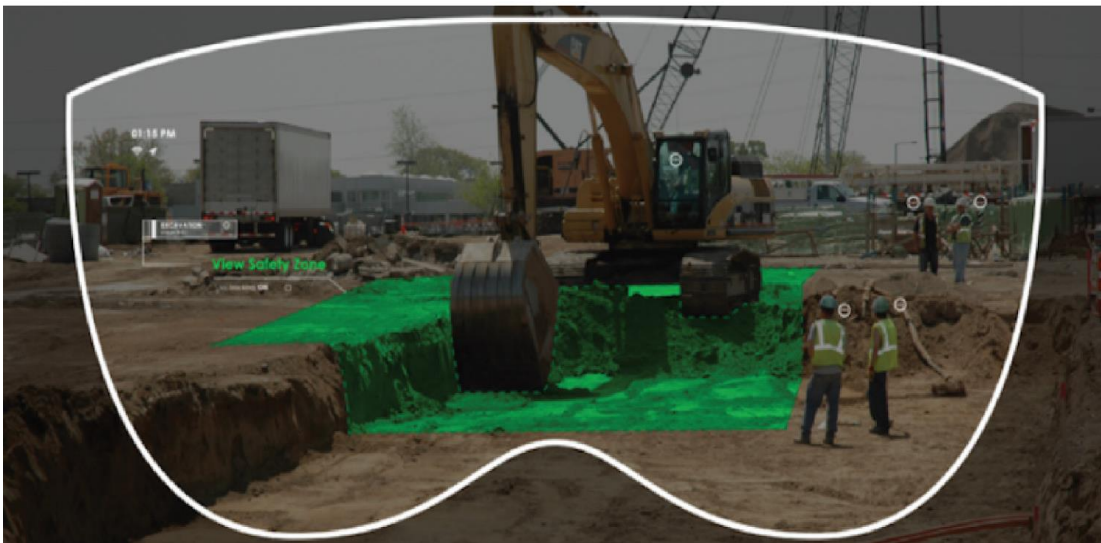
Figure 3: AR-based wearable glass for construction safety (Ahmed, S., 2019)
