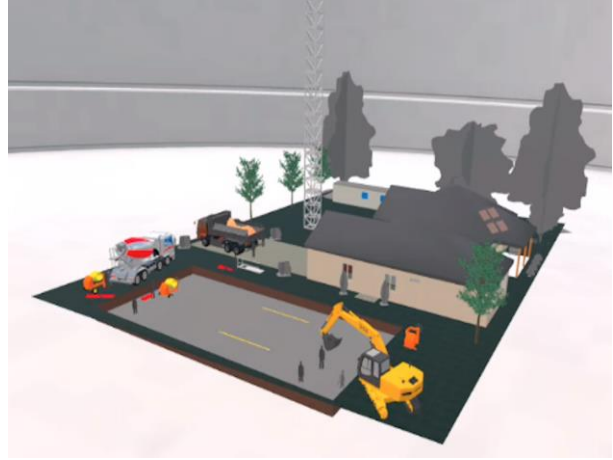
(b) Concrete works
