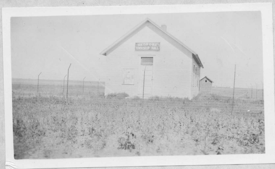
Township Hall Located in Nedrose Township, Northeast of Minot.
