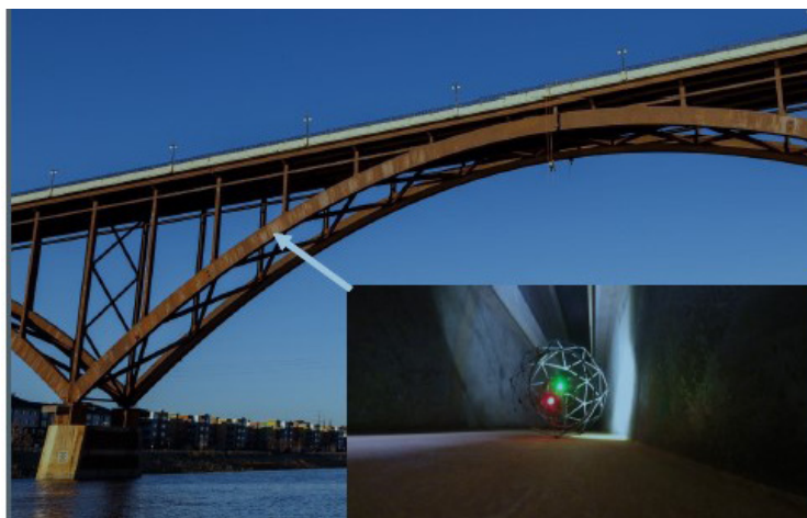
Figure 3.24 Elios conducting an inspection inside a steel box beam
