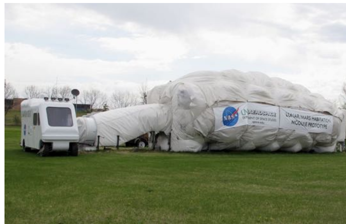
FIGURE 5. MPRS core habitat module with docking tunnel extended to the side-docking port on the lunar/Mars rover simulator. Pablo de Leon Photo credit.
