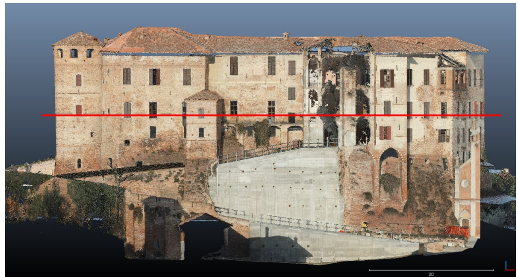
Figure 17. Profile 3 on the z axis, slicing only the castle at 11.50 m from the terrain level.
